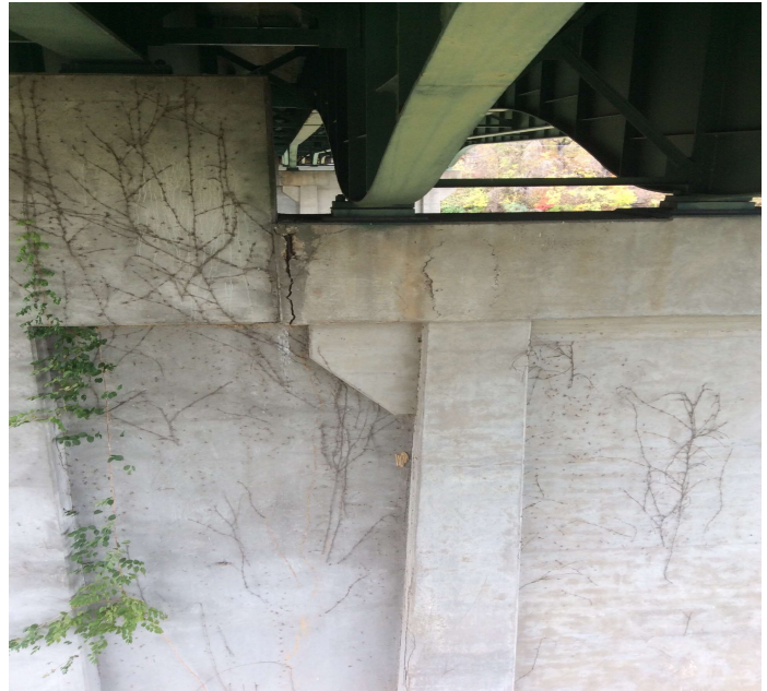
PHOTO 2 Description Spall with Rebar Exposed to Bent 5 on ahead side. Typical of random areas @ other Bents.
