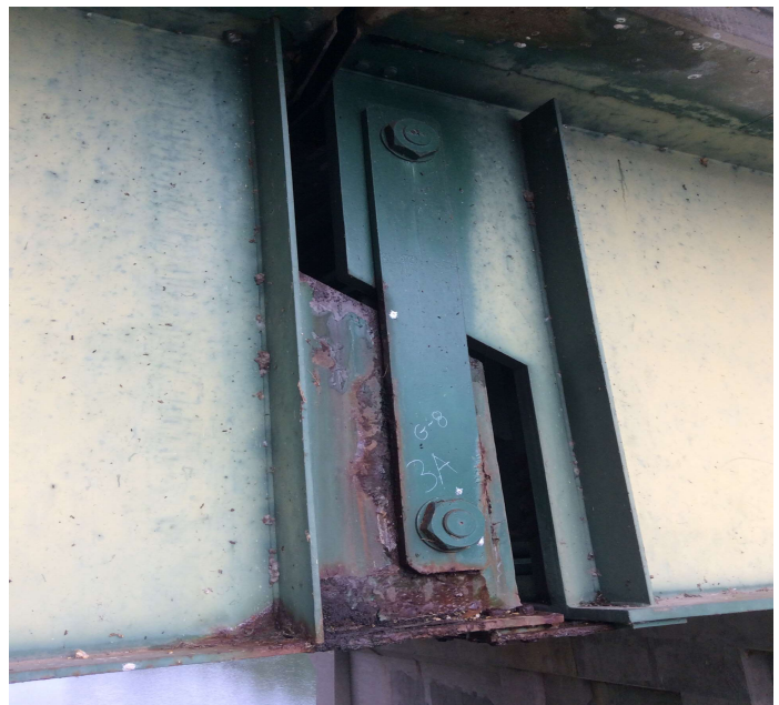
PHOTO 2 Description Typical pack rust & Section Loss to Pin & Hanger Assembly, Web of Girder, Vertical Stiffener & bottom Flange @ Span 3 Girder 8.
