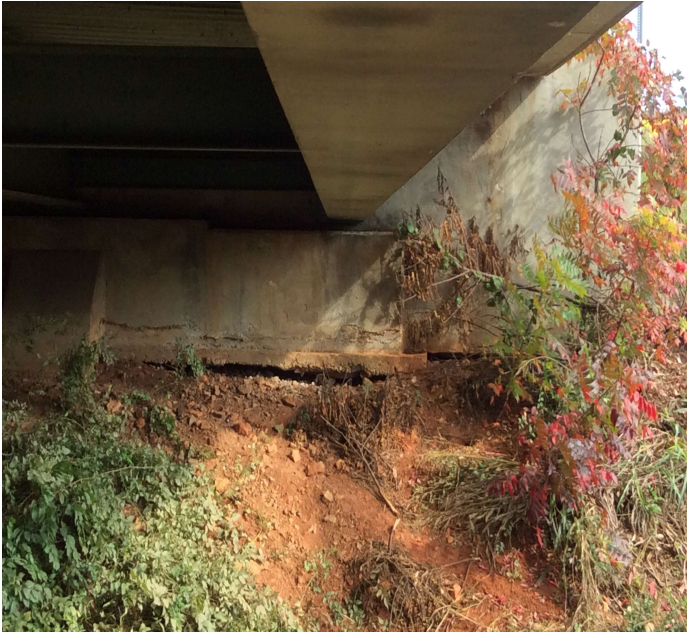
PHOTO 3 Description Erosion & Undermining to Right end of Abutment 2 with 1 Pile exposed.
