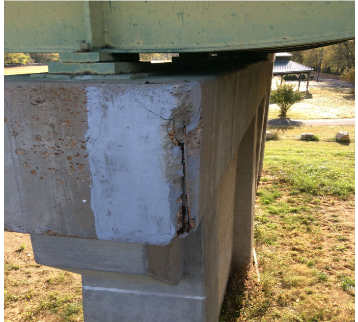
PHOTO 5 Description Left end of Cap @ Bent 5 Spall with 2' Rebar Exposed with 100% Section Loss.
