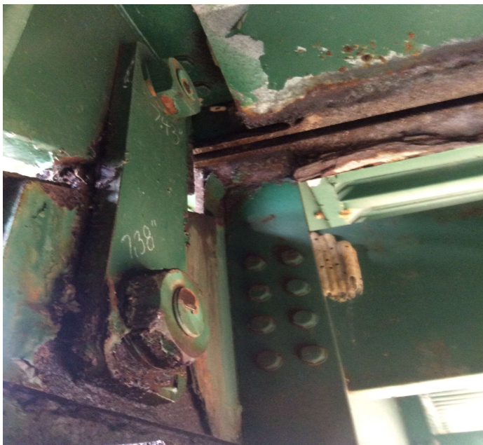
PHOTO 1 Description Typical rust, pack rust & Section Loss to Pin & Hanger Assemblies @ Girders 1 - 8 Spans 2 - 10.
