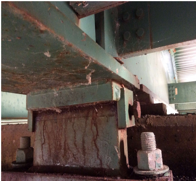
PHOTO 1 Description Bolts have backed out on Left & Right sides of Bearing Assembly 7 @ Bent 1.
