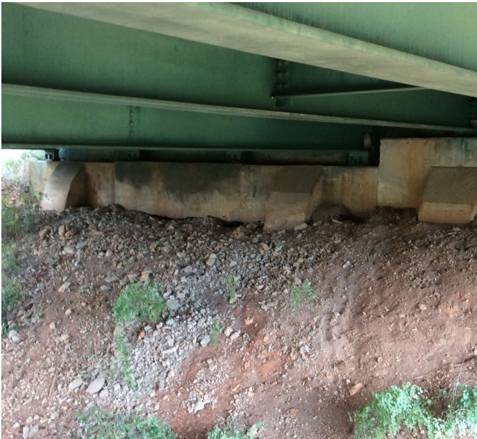
PHOTO 4 Description Erosion & Undermining to Left end of Abutment 2 with 2 Piles Exposed.
