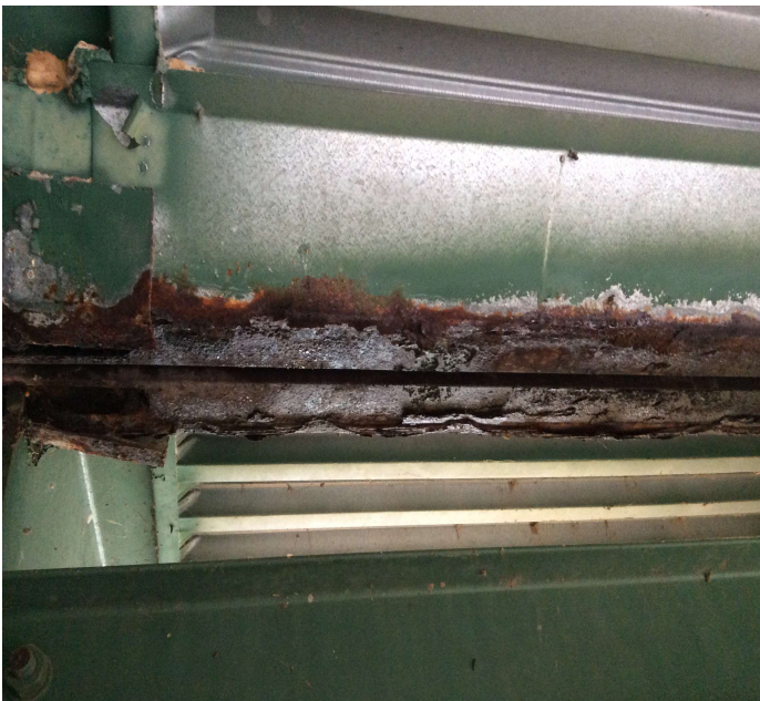
PHOTO 1 Description Heavy rust to Road Iron/Paving Haunch Assembly @ Bent 1.
