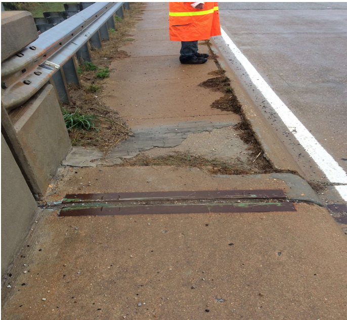
PHOTO 1 Description Sidewalk settled @ Abutment 2 on left.
