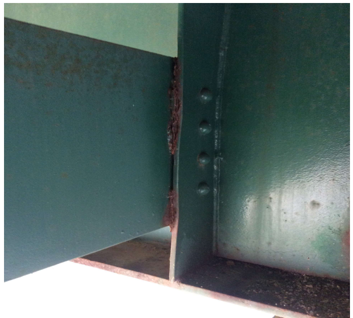
PHOTO 2 Description Typical pack rust @ Diaphragm & Vertical Stiffener Connection @ random areas.
