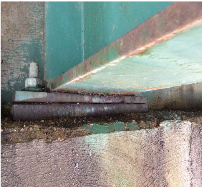
PHOTO 1 Description Typical rust & corrosion to Bearing Assemblies @ all Spans.
