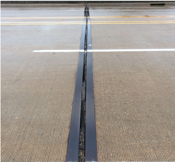
PHOTO 1 Description Typical condition of Joint Seals @ all Spans.
