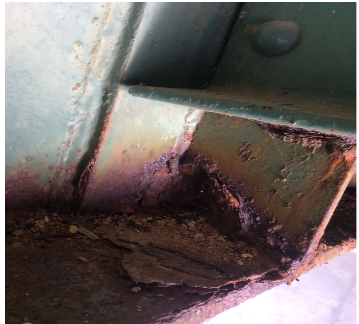
PHOTO 2 Description Span 4 Girder 3 Hole in 1st stiffener back of Pin & Hanger Assembly.
