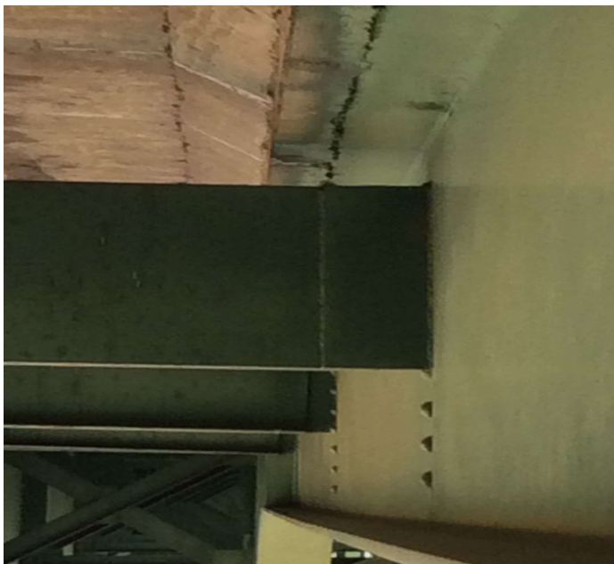
PHOTO 3 Description Cracked weld to 3rd Diaphragm ahead of Bent 9 on Left side between Girder 4 & 5 @ Span 10.
