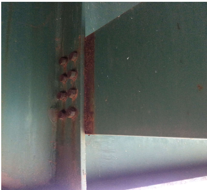
PHOTO 1 Description Typical rust to Vertical Stiffeners @ Diaphragm Connections.
