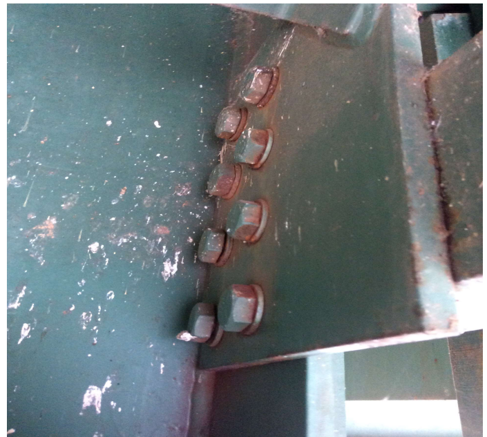
PHOTO 2 Description Loose bolts 1st Diaphragm Connection ahead of Pin & Hanger Assembly between Girder 4 & 5. Typical @ several Spans.
