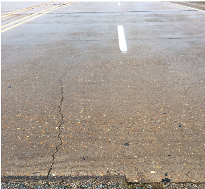
PHOTO 1 Description Moderate unsealed cracks in South lanes @ Abutments 2.
