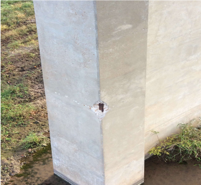
PHOTO 3 Description Typical Spall to Concrete Column 1 @ Bent 8.
