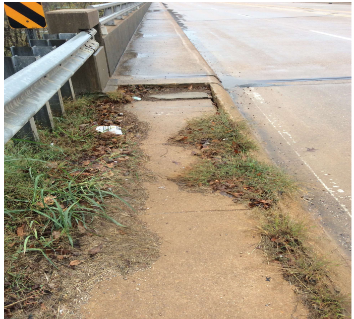
PHOTO 2 Description Settlement to sidewalk @ Abutment 2 on Right.
