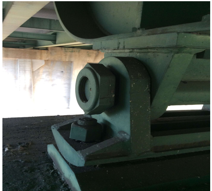
PHOTO 2 Description Nut is backed off at Bearing Assembly @ Girder 3 Bent 9.
