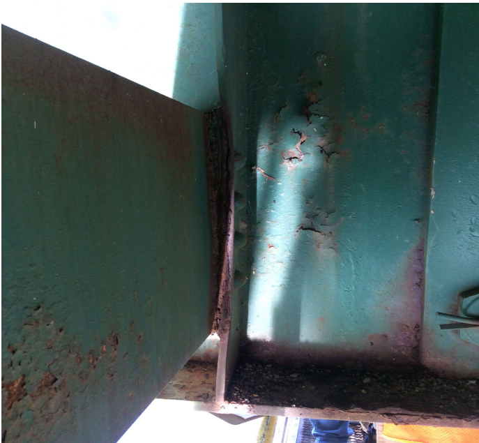
PHOTO 3 Description Span 4. Pack rust to Stiffener back of Pin & Hanger Assembly @ Girder 3.
