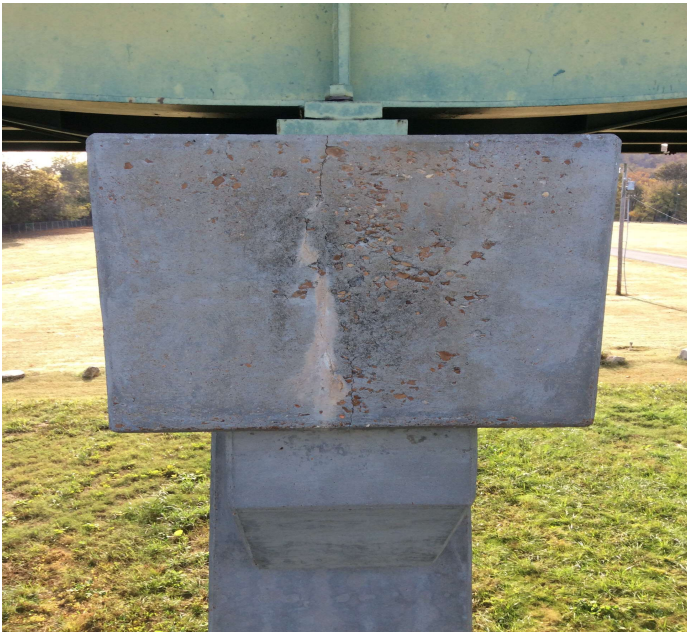
PHOTO 4 Description Efflorescent crack to Left end of Cap at Bent 7.
