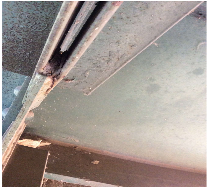
PHOTO 2 Description Diaphragm between Girder 2 & 3 @ Bent 2. Cracked weld to Diaphragm on back side.
