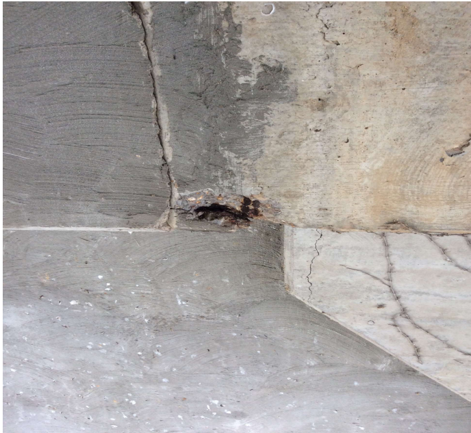
PHOTO 1 Description Typical Spall with Rebar Exposed to Concrete Caps @ random areas.
