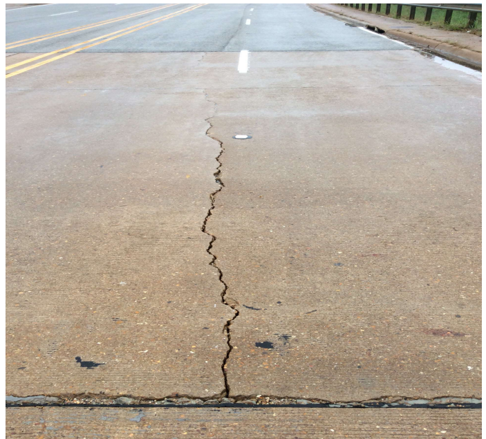
PHOTO 2 Description Moderate unsealed cracks in South lanes @ Abutment 1
