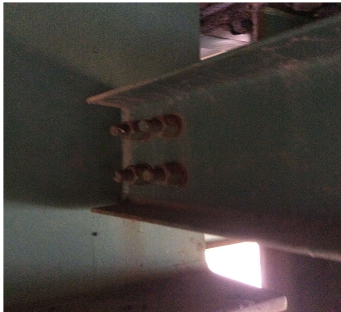
PHOTO 1 Description Loose bolts to Diaphragm Connection between Girders 4 & 5 Bent 1. Typical condition @ Spans 4 - 10.
