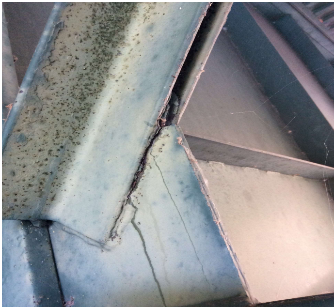
PHOTO 1 Description Diaphragm between Girder 1 & 2 @ Bent 2. Cracked weld to Diaphragm on ahead side.
