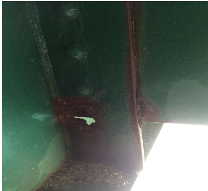
PHOTO 1 Description Hole in 1st Stiffener back of Pin & Hanger Assembly at Girder 3 @ Span 6.
